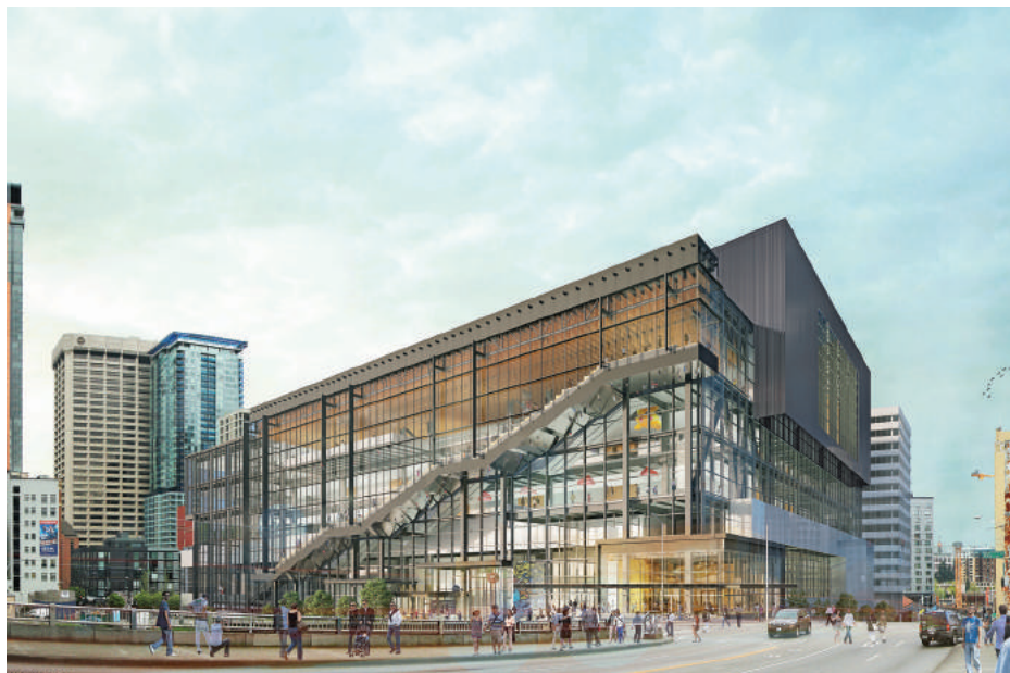
CONVENTION CENTER Construction is underway on this $960-million expansion project.
