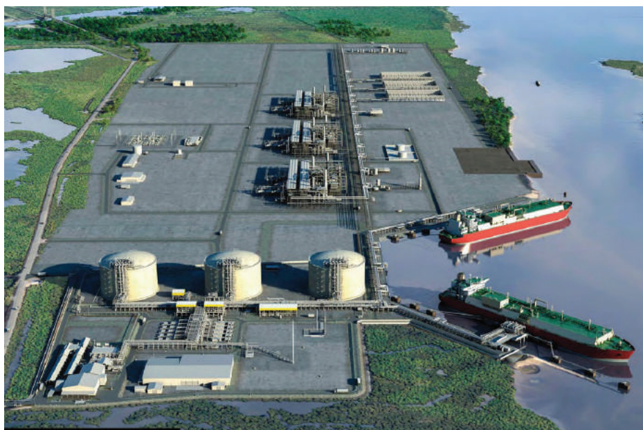
CAMERON TRAINS A rendering of an export facility being built in Hackberry, La.
