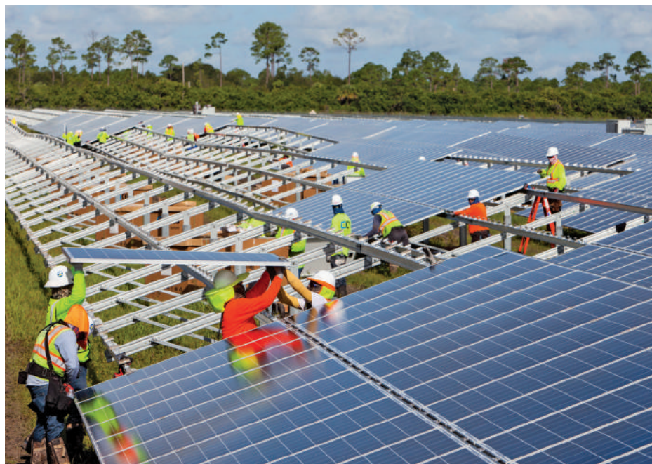
ONE OF MANY FPL is building or has built 18 solar plants throughout Florida. Black & Veatch is EPC on several.
