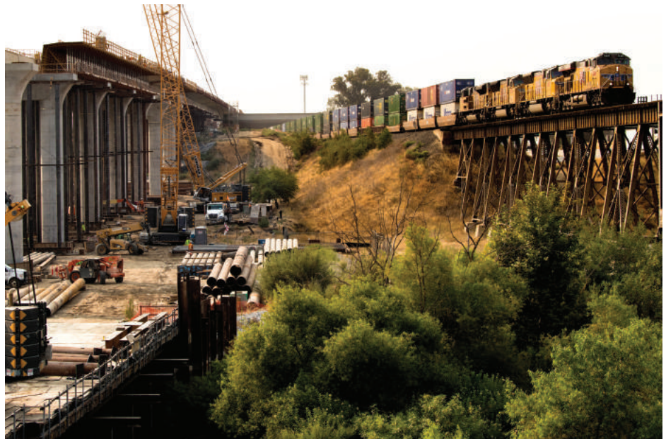
RISING HIGH Precast girder viaducts parallel existing active railroad as part of $3 billion in high-speed rail work.
