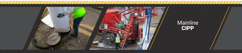
In addition to continual monitoring of temperature readings at boiler trucks, our team has implemented new fiber optic monitoring technology. Where earlier efforts provided readings at intervals of 200 to 300 feet using thermocouple measuring devices at manhole access locations, our thermal imaging system now enables the monitoring of the curing process along the entirety of the pipe run at 6-inch intervals.
