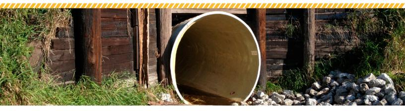
Our most widely used solution is our proprietary Inliner® Cured-in-Place Pipe. CIPP is a proven, cost-effective no dig solution for problems normally associated with leaking or deteriorated pipelines.
