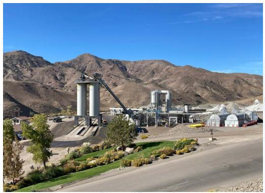
Installing warm-mix asphalt systems to allow asphalt production at lower temperatures to reduce energy use—Granite was an early adopter of these systems, and has retrofitted 28 asphalt plants to produce warm-mix asphalt
